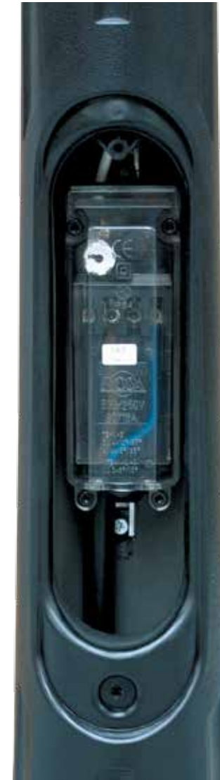
Connection box installed in plastic coated pole
