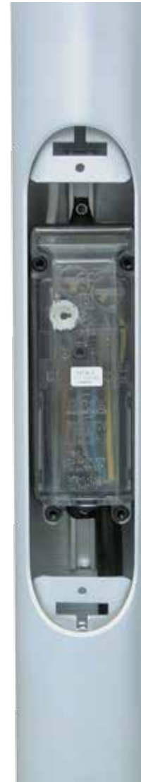
Connection box installed in aluminium column
